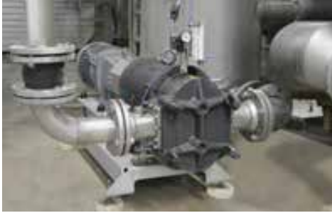
ONIXline pump for conveying C starch
