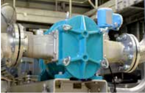
BLUEline pump for conveying cleaning agent
